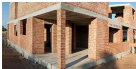
**Figure1.** Load bearing masonry wall
