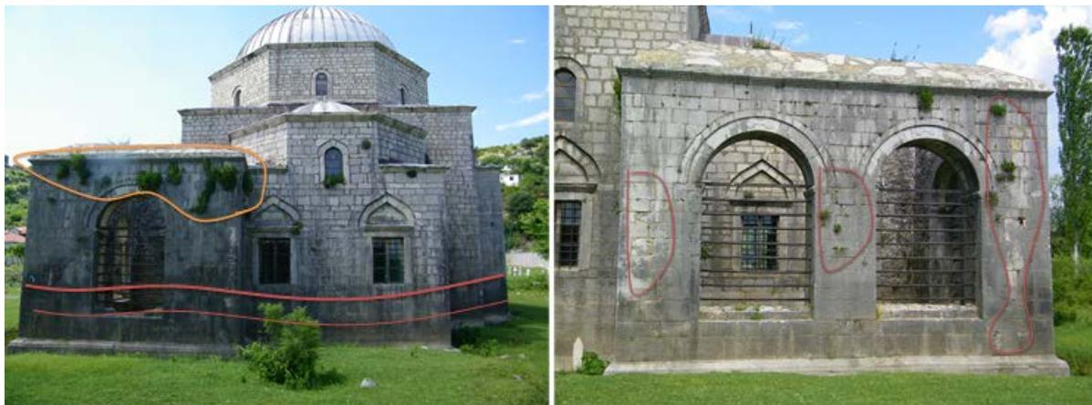
**Figure 4.** Traces of weathering factors influence and acceleration biological degradation in Lead Mosque
